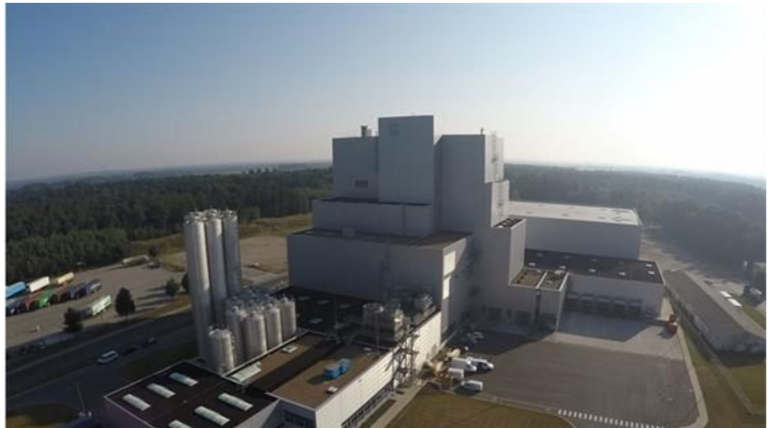
Example of a spraying tower
